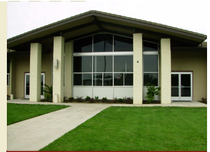
SSJID's Main Office will soon be able to utilize water from the City of Manteca with the construction of a new water line connection to the city's Austin Road pipeline.
