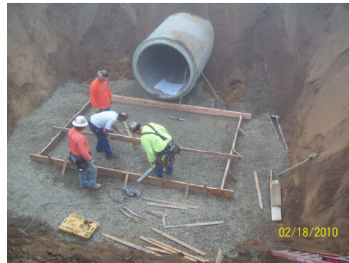
A crew from Clyde Wheeler Pipeline forms the floor for a box on the Lateral R in Manteca, a pipeline replacement project north of Louise Ave. between Austin and Prescott Roads.
