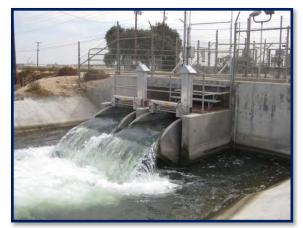
Figure 3-6. Flume Gates at Lateral Heading
