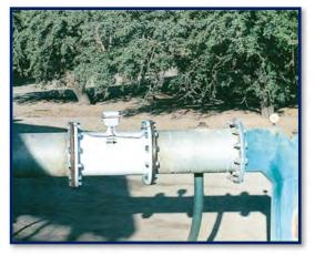
Figure 3-16. Magnetic Flow Meter
