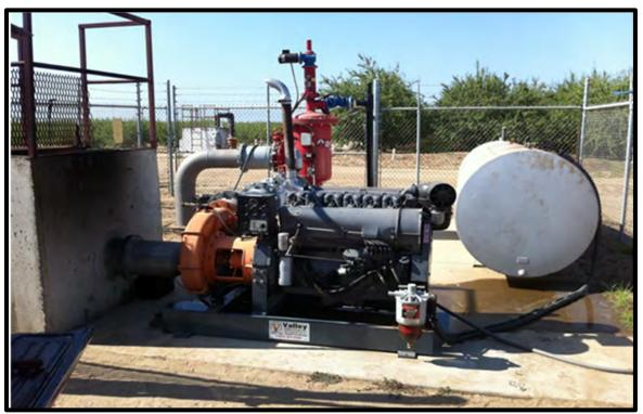
Figure A-2. Pump turnout on a District pipeline.
