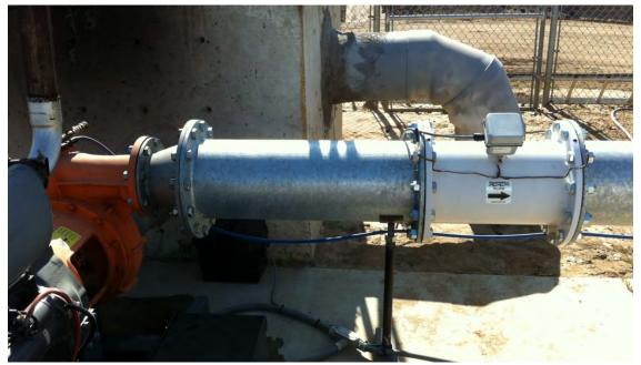
Figure A-6. Magnetic flow meter on delivery at Ra81.
